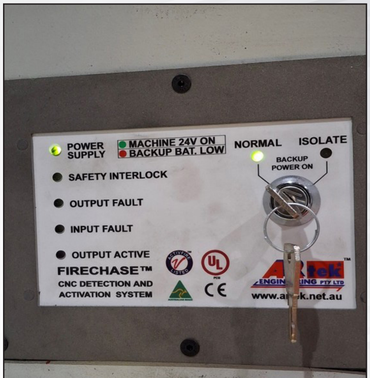
FIRE SUPPRESSION SYSTEM ACTIVATE/DEACTIVATE
